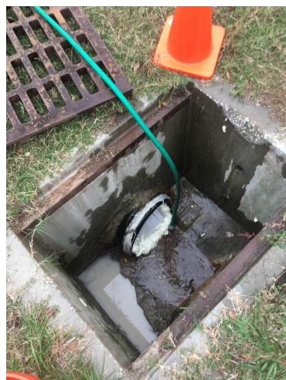
Figure 7. Drain line partially plugged and filled with pyrethrin-treated water.
