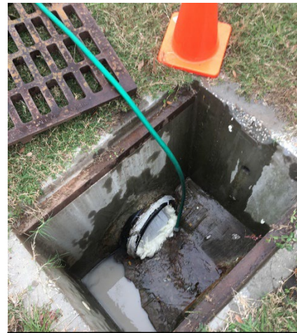
Figure 3. Drain line partially plugged and filled with pyrethrin-treated water.
