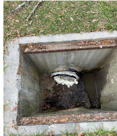
Figure 3. Access well with partially plugged drain line.
